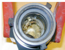
Actual Attack Nozzle A bird nest, 3 birds and a tennis ball entered an unprotected FDC clogging the backup fire line.
