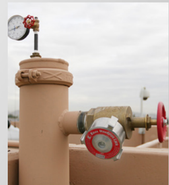
Knox Standpipe Lock on a roof top standpipe
